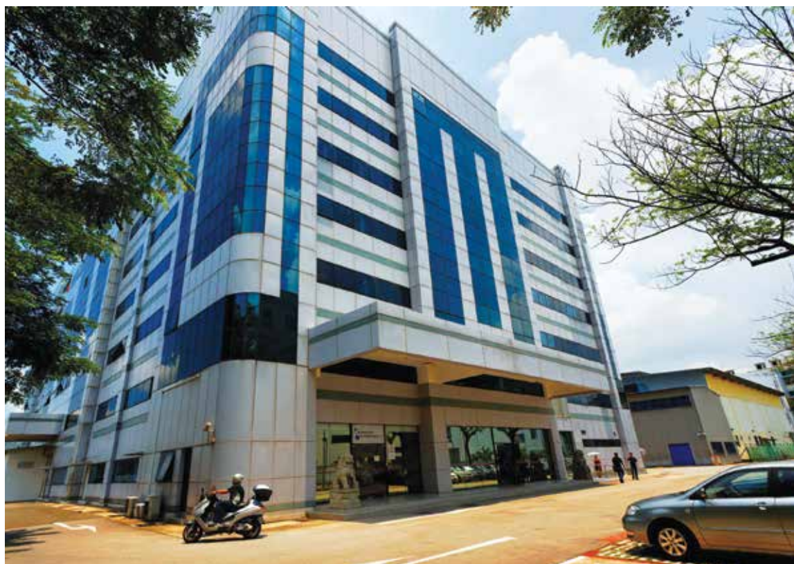
Light Industrial Building, 26 Woodlands Loop
