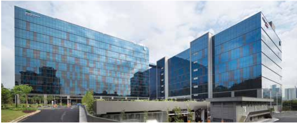
Hi-Tech Buildings, 1 and 1A Depot Close
