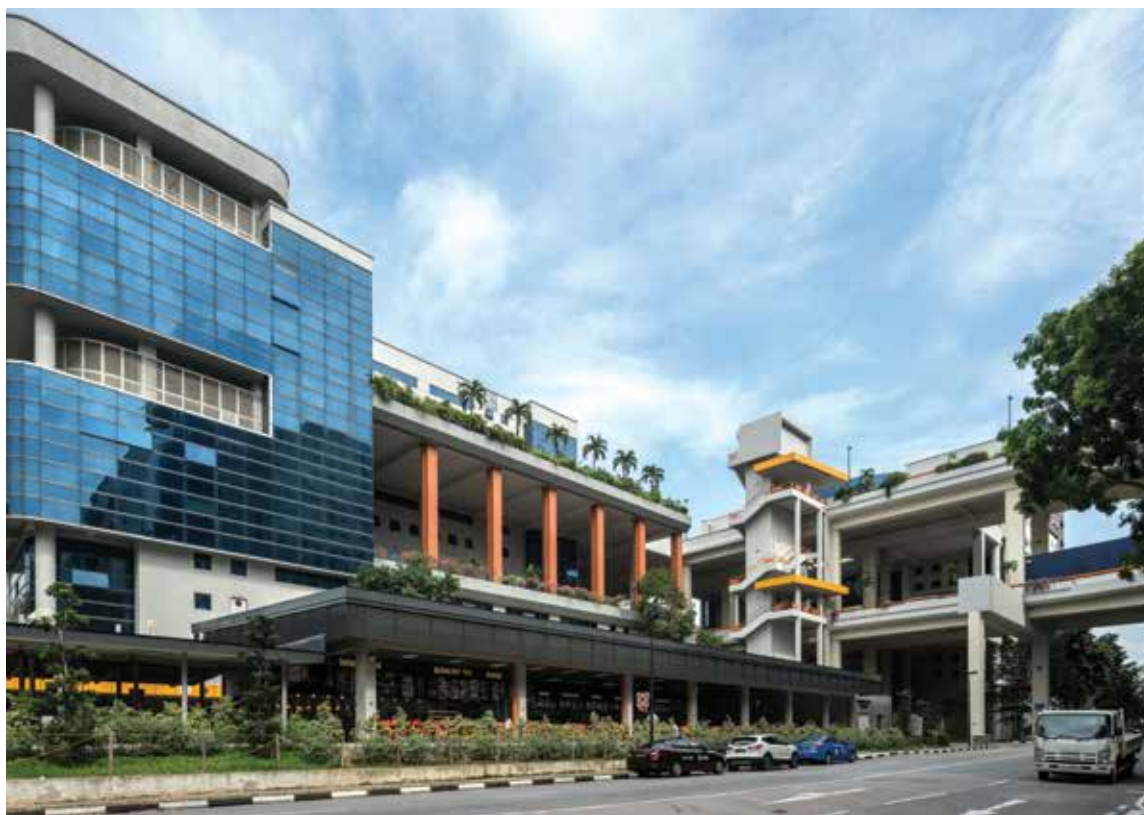
Stack-up/Ramp-up Buildings, Woodlands Spectrum
