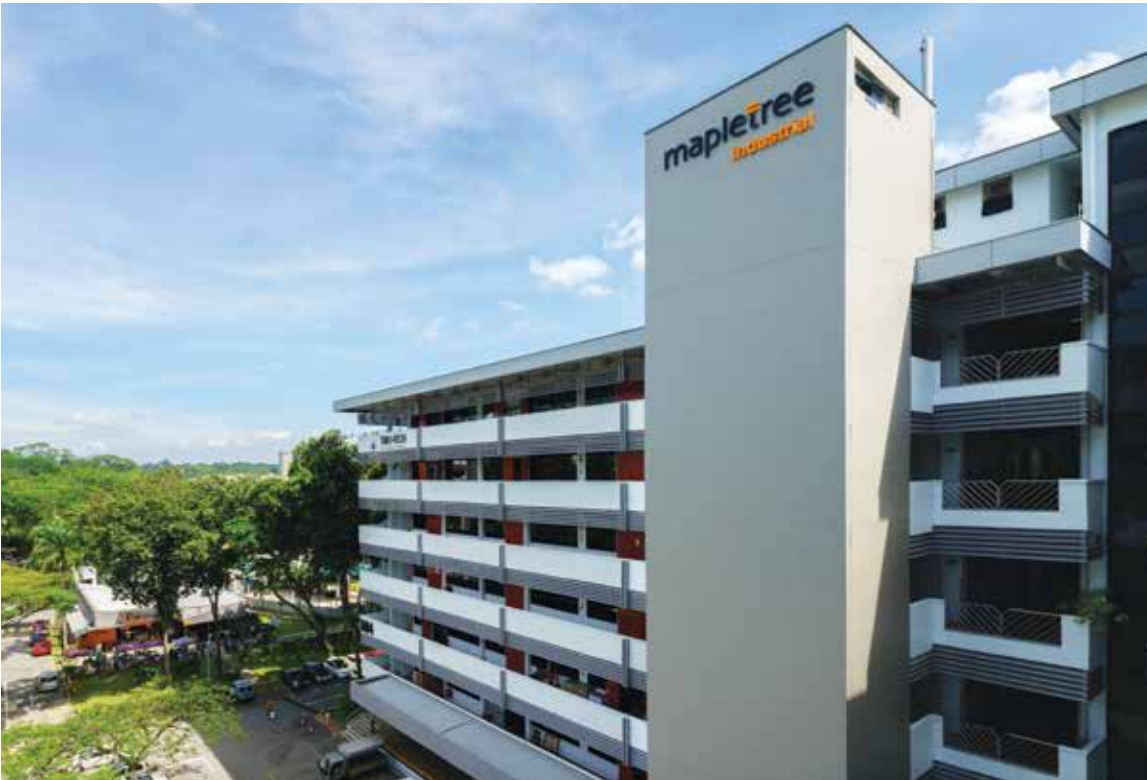
Flatted Factory, Toa Payoh North 2
