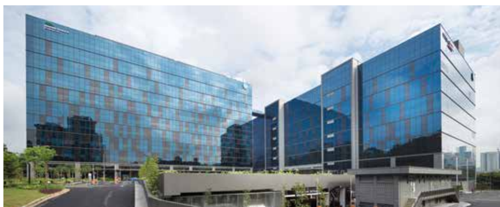
Hi-Tech Buildings, 1 and 1A Depot Close
