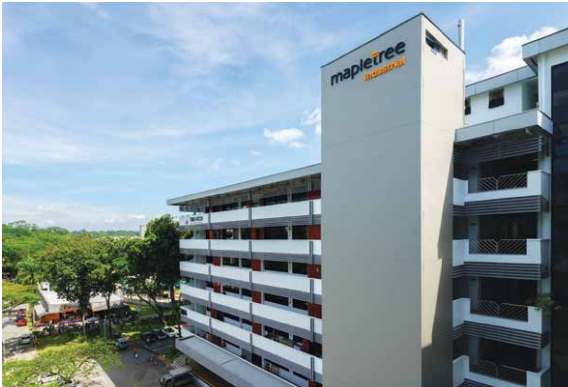
Flatted Factory, Toa Payoh North 2
