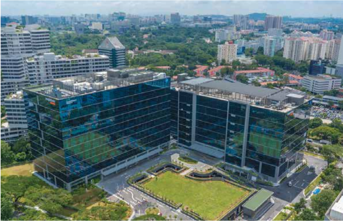
BTS facility for HP at Depot Close.
