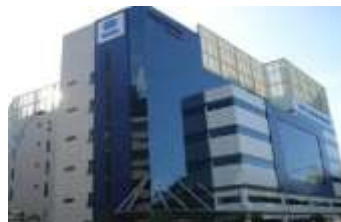
Light Industrial Buildings
