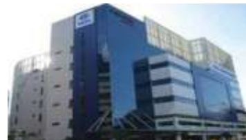
● Tata Communications Exchange
