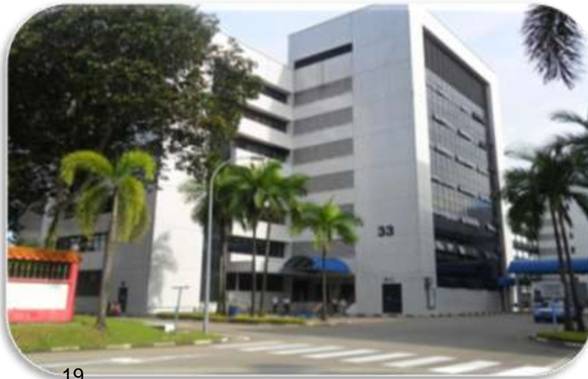
Woodlands Central Cluster before redevelopment
