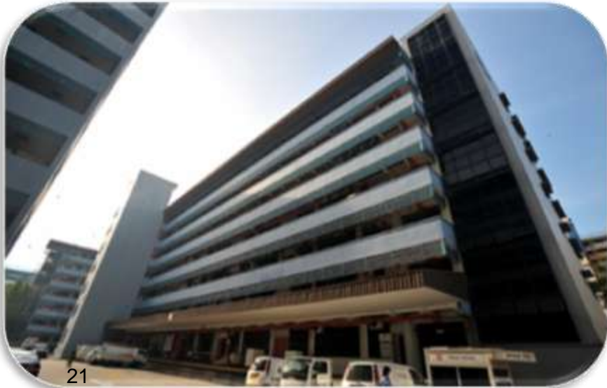
Toa Payoh North 1 Cluster before redevelopment
