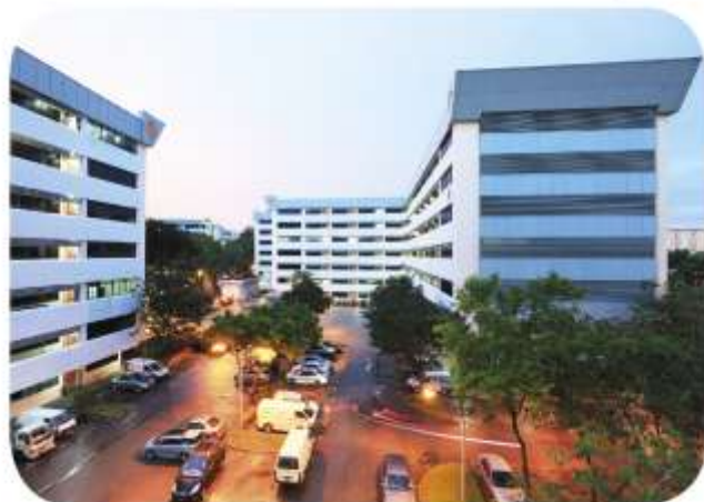
Flatted Factory, Kallang Basin 2
