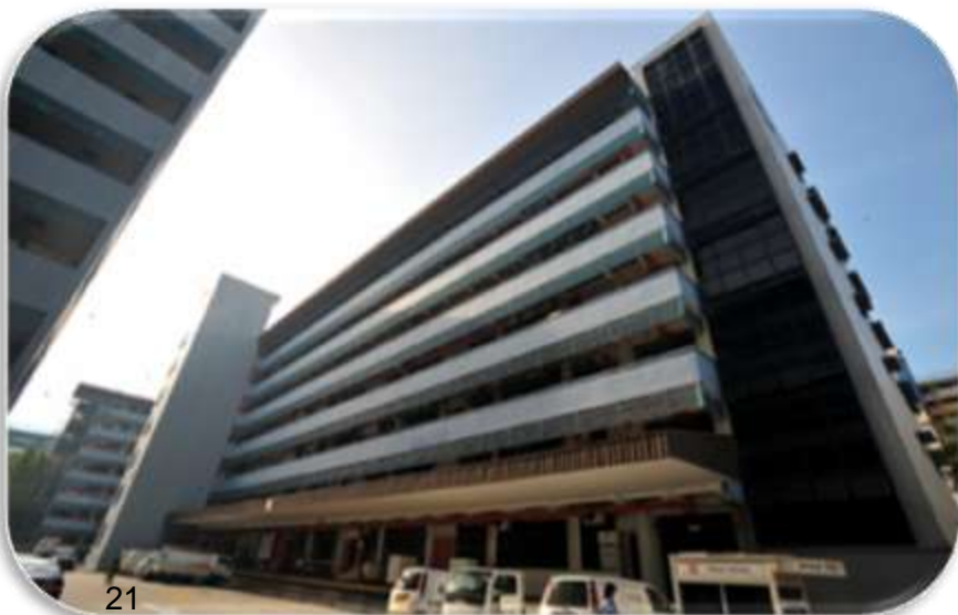
Toa Payoh North 1 Cluster before redevelopment
