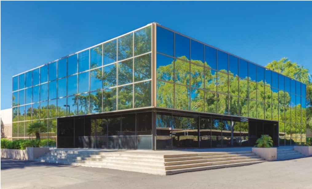
2601 West Broadway Road, Tempe located in Arizona, the US, is part of the Group's growing portfolio of data centres.
