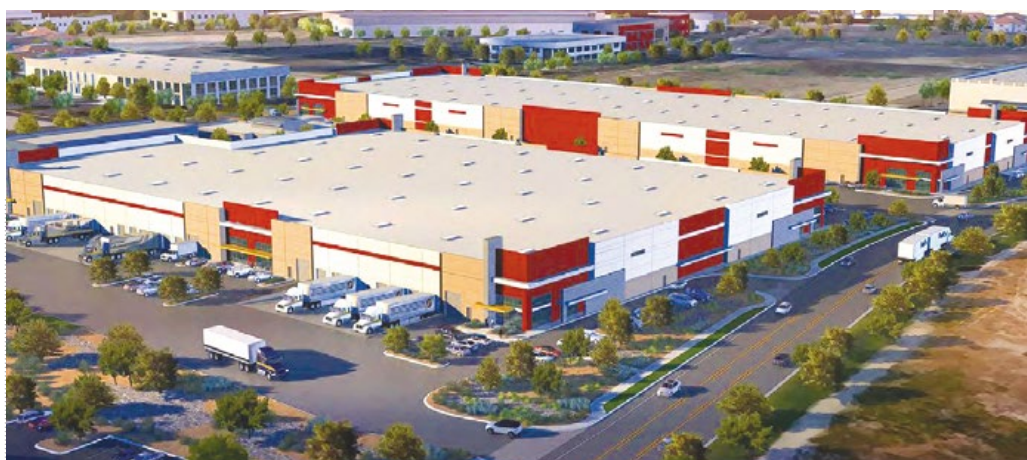
South Valley Building A consists of a single warehouse block fully equipped with fire sprinkler systems, and offers a 32-foot ceiling height, 134 parking spaces, 28 dock doors and four drive-in doors.
