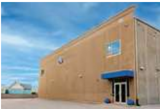
21 505 West Merrill Street, Indianapolis
