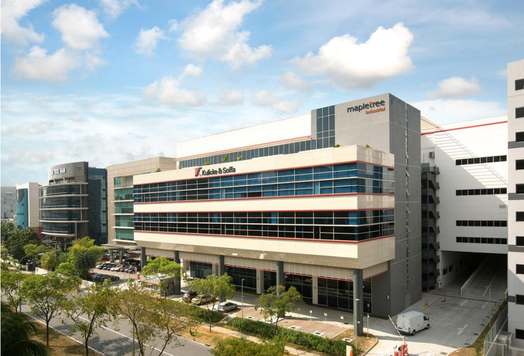
K&S Corporate Headquarters (Build-to-Suit Project by Mapletree Industrial Trust)
